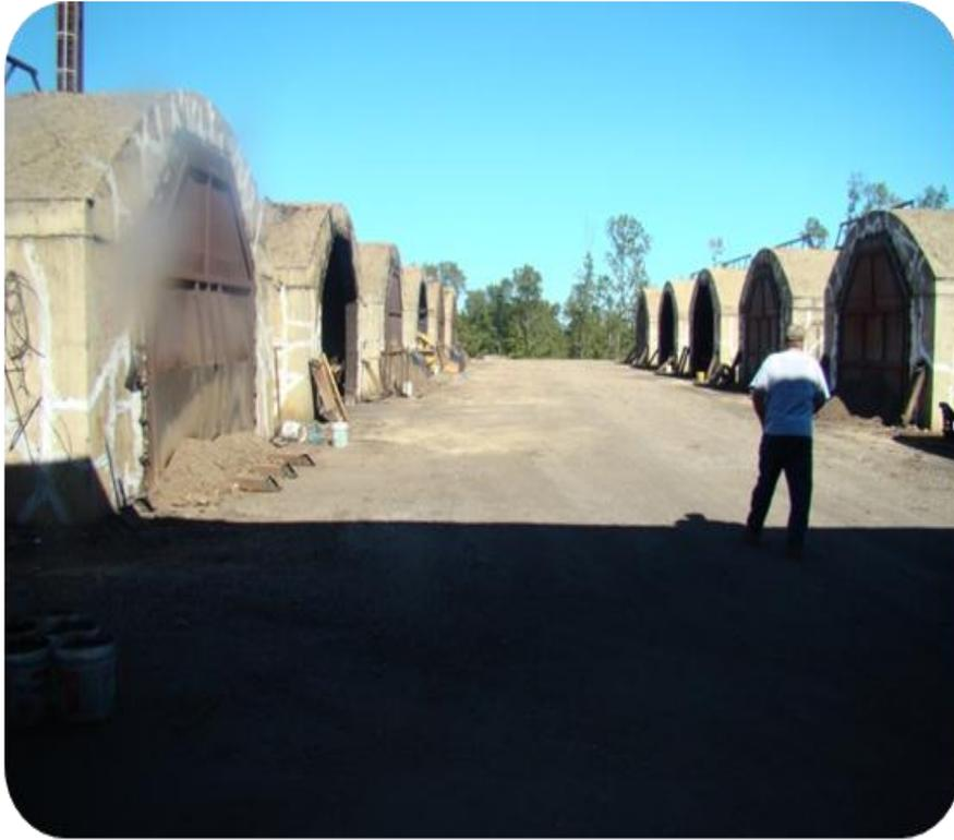
**These are some of the kilns located in the heart of Missouri where the Good-One™ charcoal is produced. The wood used is primarily scrap from saw mills mixed with some cordwood, often remains from trees cut for saw logs or wood staves.**
