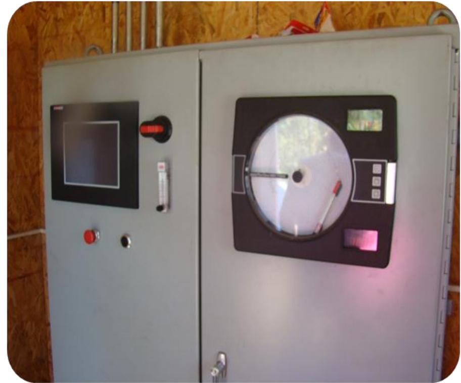
**This is the computer control room (about \$60,000 worth) which is used to control the afterburner. Below is a graph recorder for the afterburner which is monitored around the clock by the Department of Natural Resources.**
