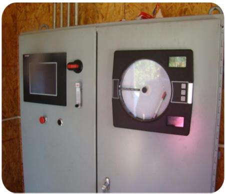
This is the computer control room (about \$60,000 worth) which is used to control the afterburner. Below is a graph recorder for the afterburner which is monitored around the clock by the Department of Natural Resources.
